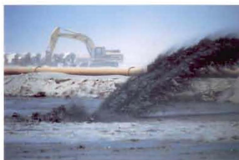
Pipeline end of land reclamation
