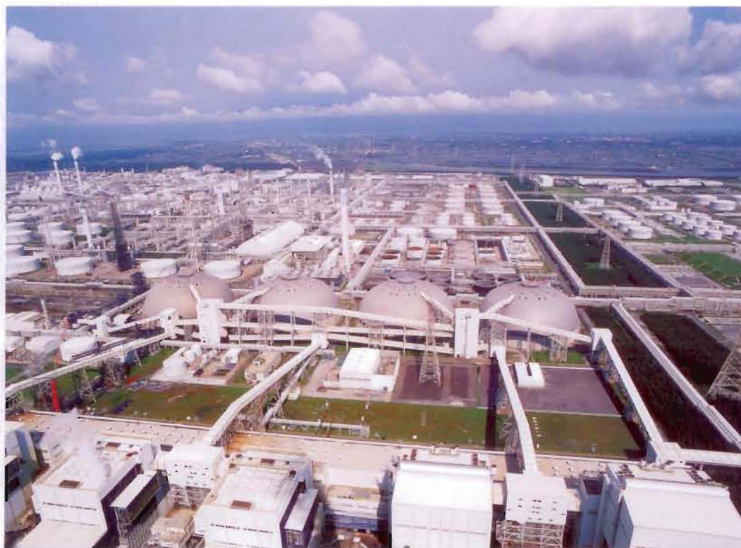
All plant areas are installed with automated closed coal bunkers to eliminate flying dust and protect the air.
