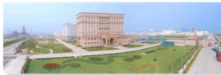
Ningbo Factory in China
